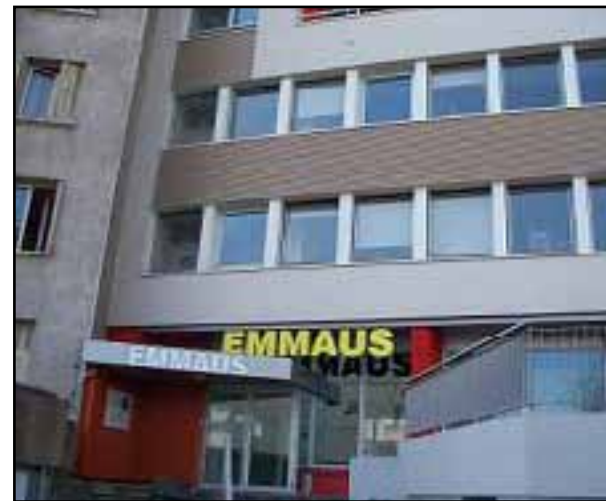
Emmaus Headquarters in France
