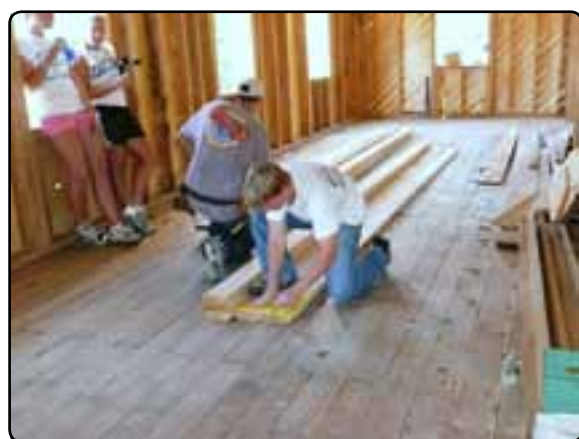
Volunteers from Madison CT, working on the Farmhouse in Dedham.
